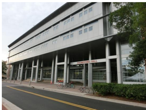
Figure 1. Engineering Hall with Abbott laboratory.
