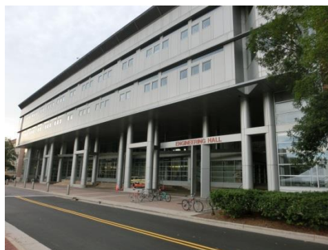
Figure 1. Engineering Hall with Abbott laboratory.
