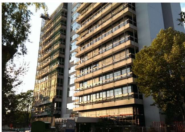
Figure 1. University of Freiburg, the building for chemistry and biochemistry
