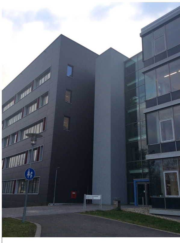
Figure 1. Newly built chemistry department building.
